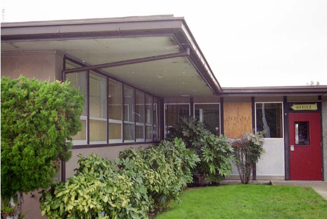
Figure 6: South Classroom Building, north face at entrance
