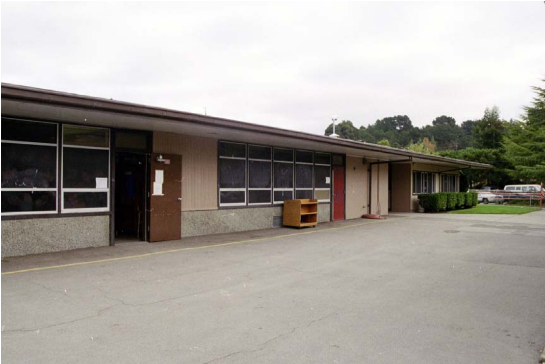
Figure 3: South Classroom Building, south face
