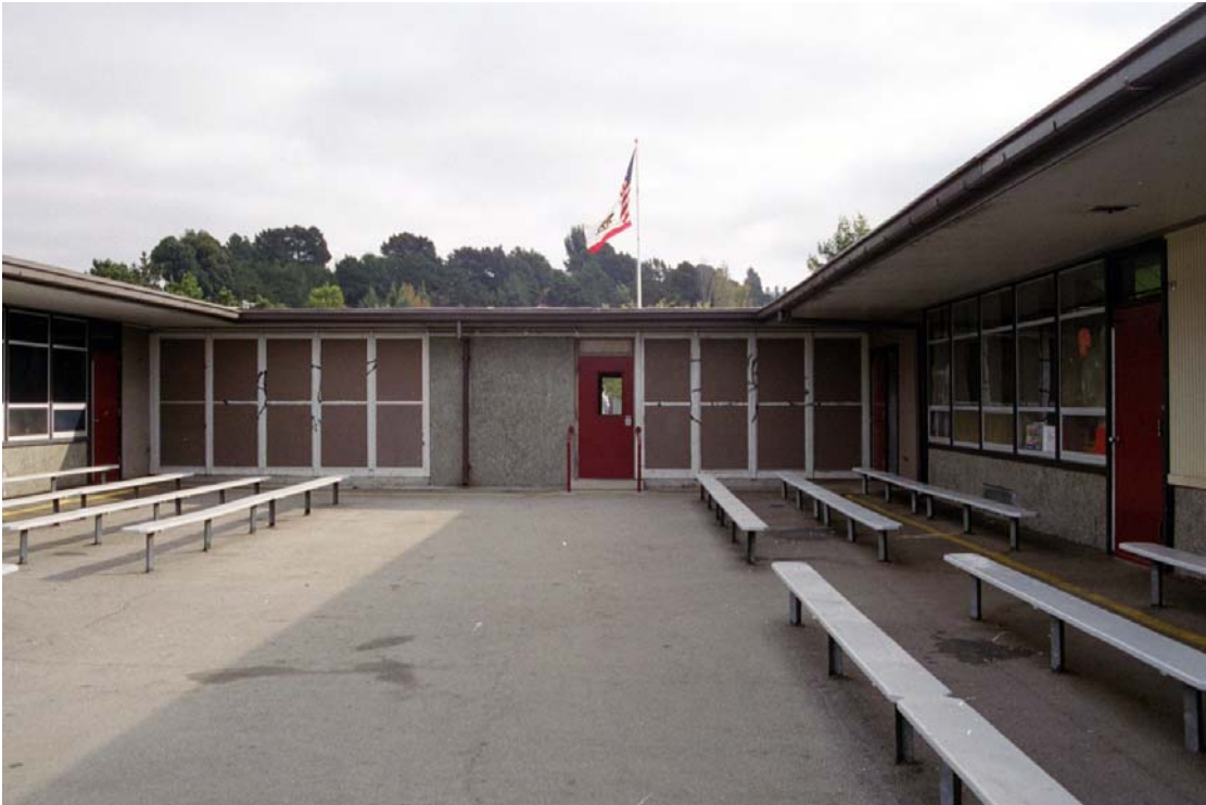
Figure 5: Enclosed Hallway, west face
