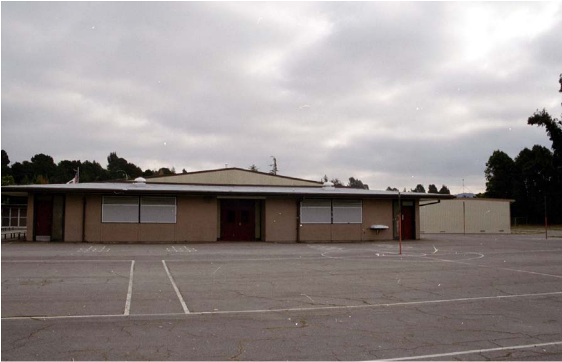
Figure 7: South Classroom Building, west face
